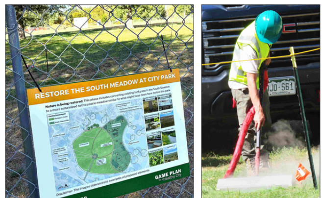
Left: Concept plan sign on temporary fencing for prairie restoration work at Denver City Park. Right: Edaphic Solutions worker steam-kills turf in project to convert a City Park meadow to shortgrass prairie (Patrick O’Driscoll)
